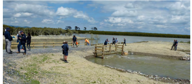
Floodgate Piako River KEITH WOODLEY
