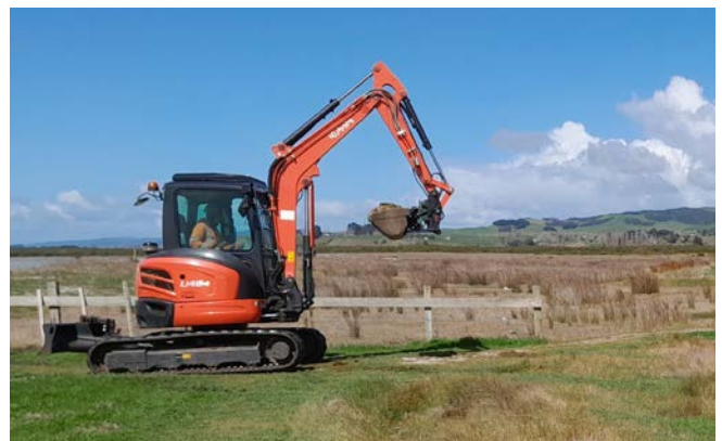
Digger work at Pūkoro Robert Findlay Reserve TANSY BLISS
