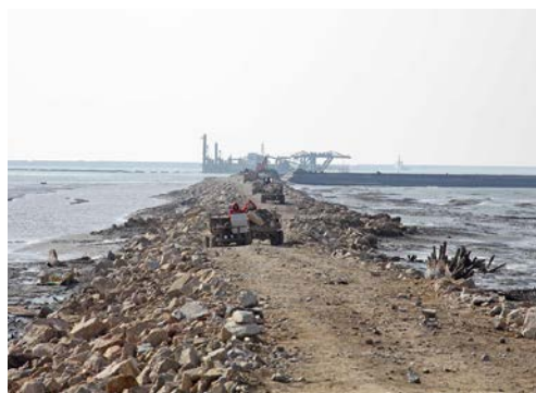
Development underway Bohai Bay China ADRIAN BOYLE.
